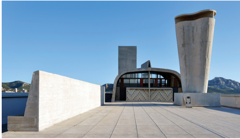
The rooftop of Cité Radieuse, Marseille Modular Arts Centre. Photo © Olivier Amsellem.
